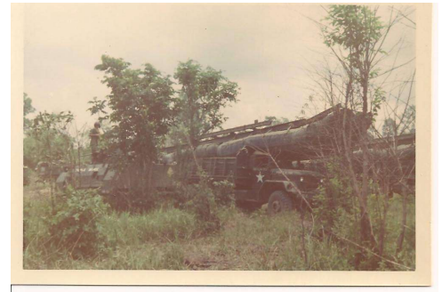
Getting the bridge ready.jpg (1008x688)
